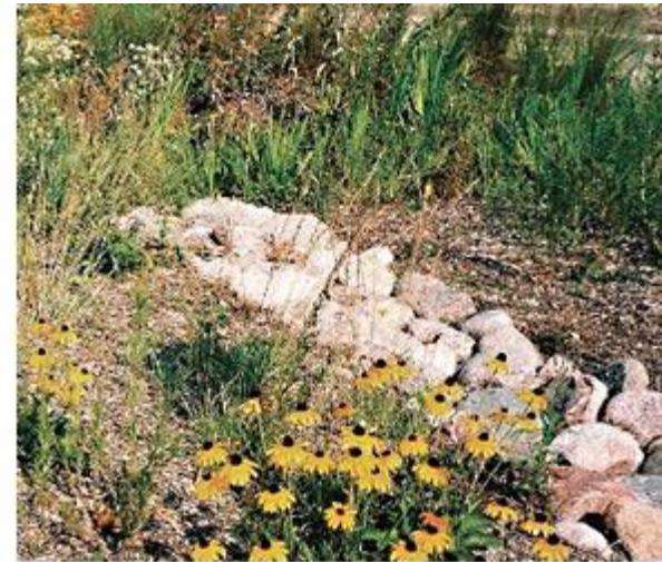
An example of a drainage swale near a parking area at the Chicago Center for Green Technology.
