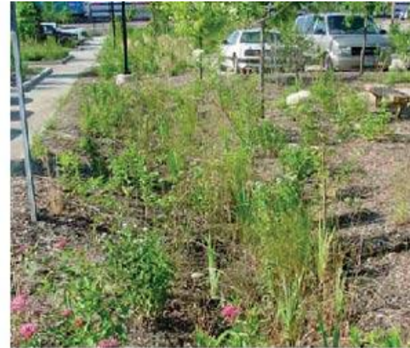
The Chicago Center for Green Technology uses filter strips to convey runoff on-site.
